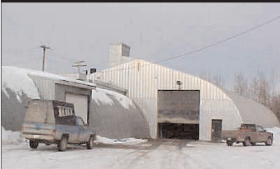
Exterior Shot of Warehouse Heated With Hot Exhaust Gas From Generator
