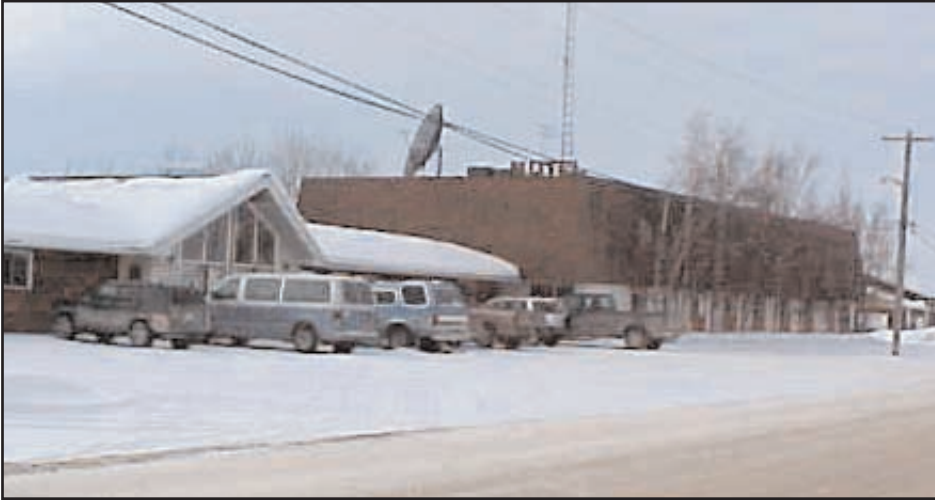
(Left to right) Residence, Office and 35-Room Motel whose Heat and Hot Water are Supplied by the Hot Water Produced by the Co-gen System
