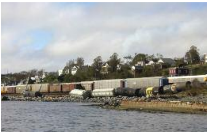
Figure 5. Aftermath of Hurricane Juan in Halifax Harbour: waves propagating up the harbour at high water undermined the outer track of the Canadian National rail yard along the Dartmouth waterfront, toppling rail cars and sending some into the harbour.
