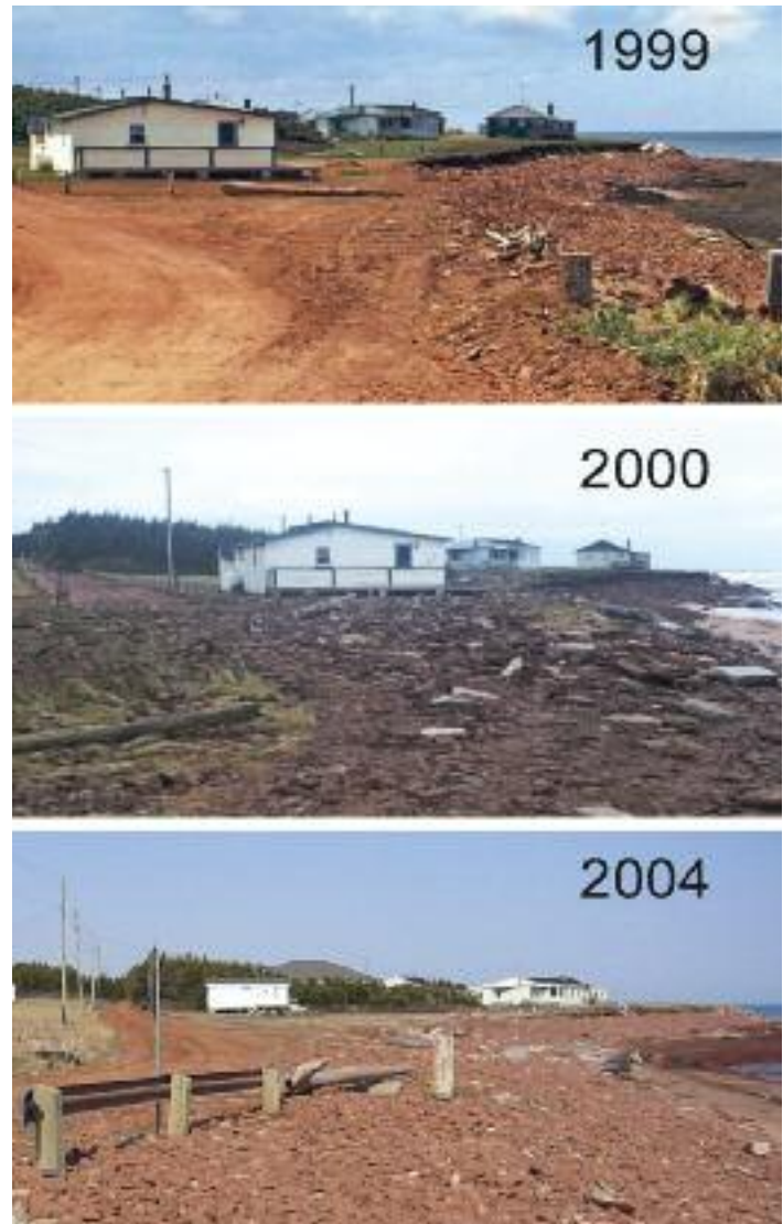
Figure 7. Time sequence shows erosion threatening cottages in 1999 and 2000 followed by severe damage and removal of two cottages by 2004, North Shore, Prince Edward Island
