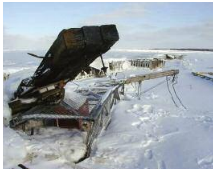
Figure 4. Navigation infrastructure was destroyed by ride-up of ice 40 cm thick during storm of January 21, 2000, in Robichaud, New Brunswick - photo courtesy of Michael Campbell, Environment Canada.
