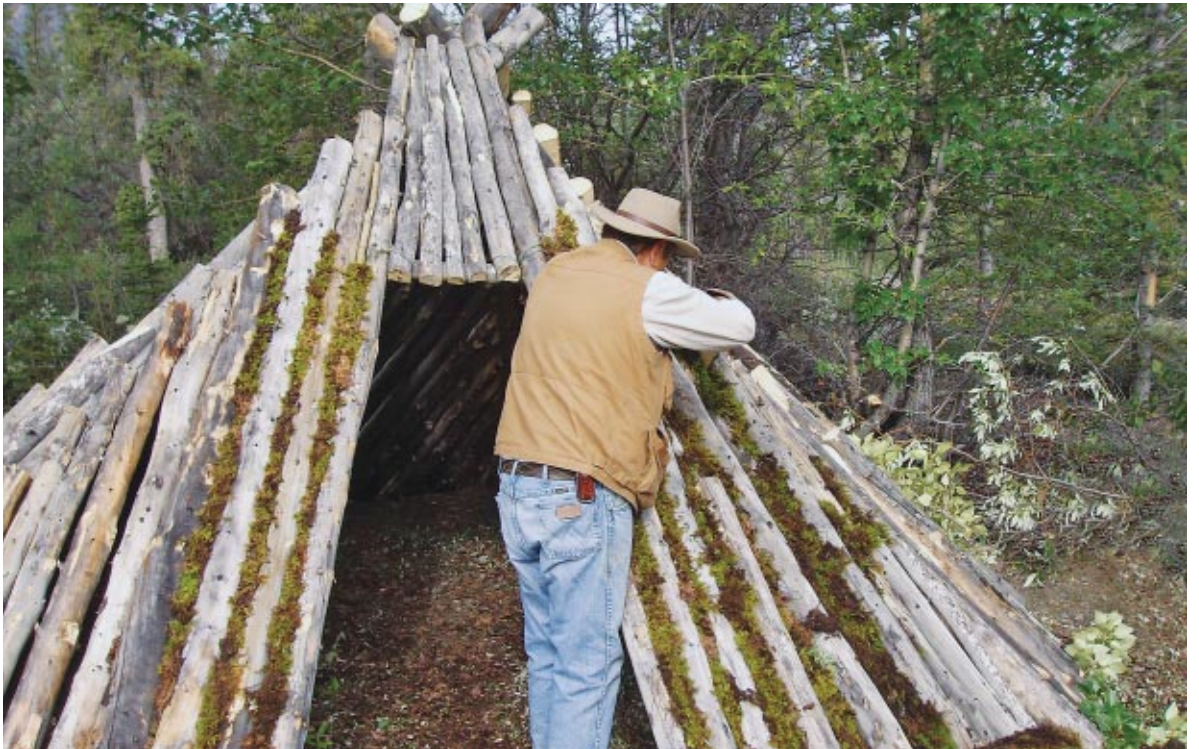
Champagne and Aishihik First Nations Elder Chuck Hume applying moss between the poles of the njäl.
