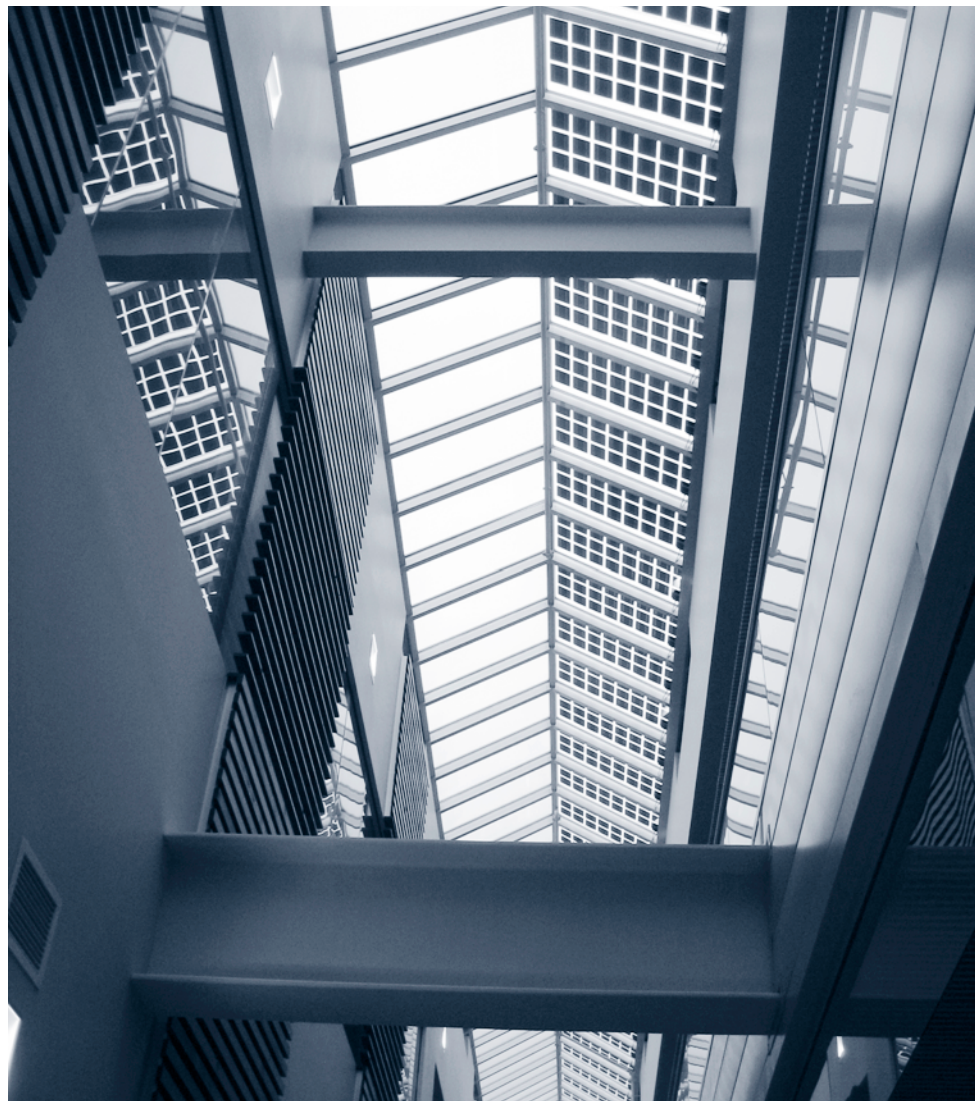
Lining the top of the facility's atrium skylights are 93 photovoltaic panels that turn solar energy into electrical power.
