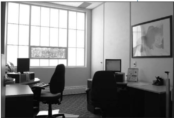
Figure 1. East room translucent sandwich panel installation. The photo was taken at noon on a sunny, mostly clear-sky day.
