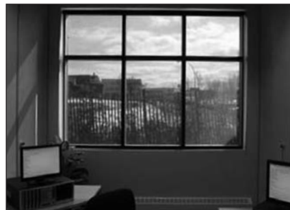
View of outdoors through a double clear window with an interior black perforated screen under a partly cloudy sky
