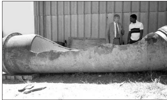
A failed large-diameter water main
