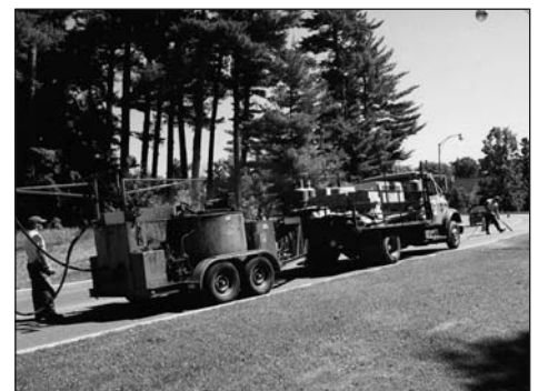
Typical crack sealing train
