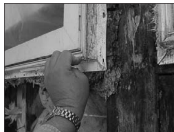
The effects of water leakage around windows
