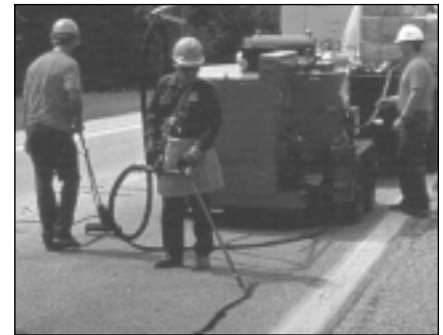
Workers apply crack sealant to pavement
