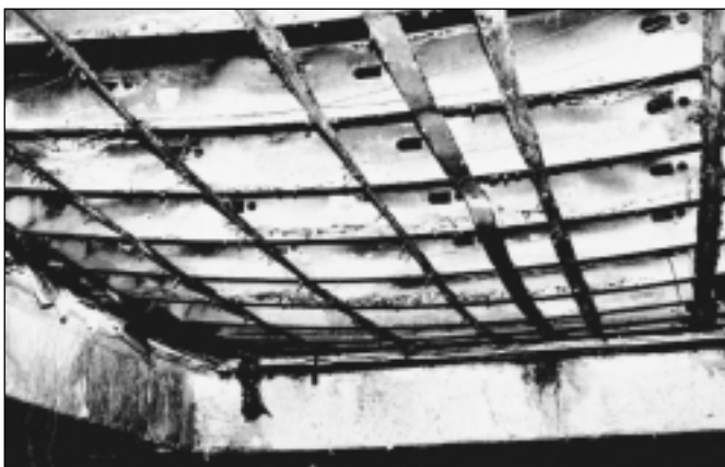
LSF joists after fire test
