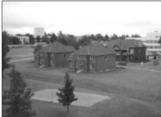
Twin research houses at the Canadian Centre for Housing Technology
