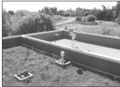
NRC's Field Roofing Facility shortly after construction. The median divider, where the weather station is located, separates the green roof (lower) from the reference roof (upper).
