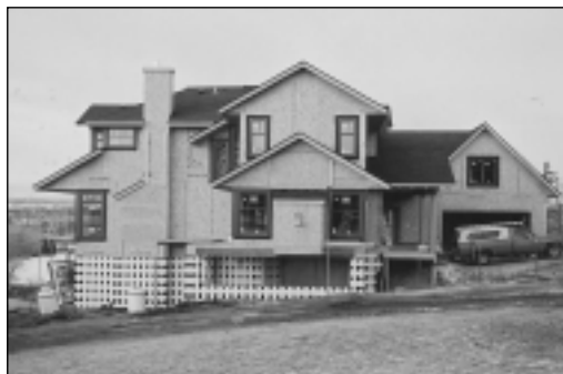
Stressed skin panels with structural ribs are used for both walls and roofs in these houses.
