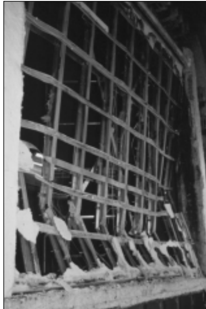
Load-bearing steel-stud wall assembly after fire test
