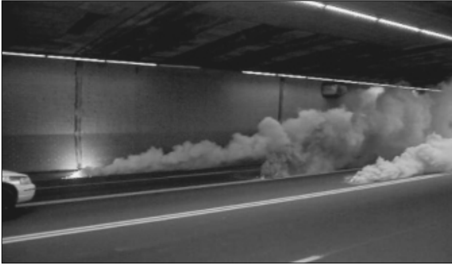
Smoke moves through a Montreal tunnel in an MTQ study of ventilation strategies in emergencies.
