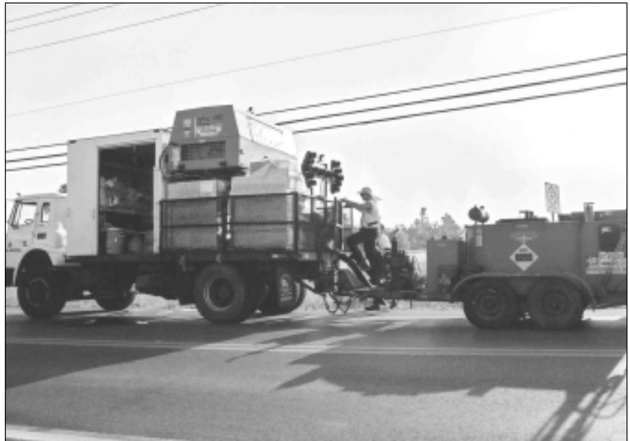
A crack-sealing train with the lead truck pulling the melter
