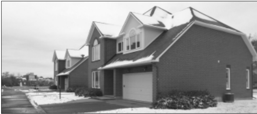
The RHT index can be used to assess the moisture performance of the building envelope in buildings such as these.
