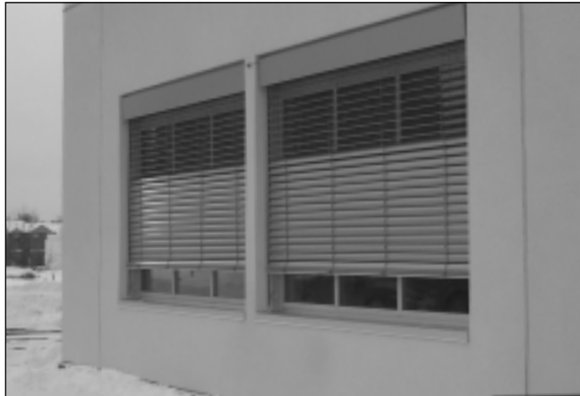
Outside view of daylighting laboratory showing the external split blind system with the slats closed in the lower part, to block direct sunlight, and open in the upper part, to admit daylight deep into the space.
