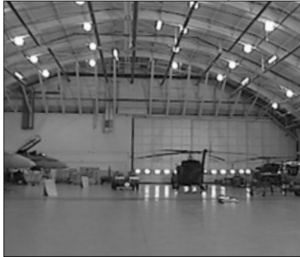
Fire researchers at IRC are studying the capabilities of various modelling tools to predict smoke movement in different types of building. The aircraft hangar, which is very large (in both area and height), but also relatively simple, is one of the building types being investigated.
