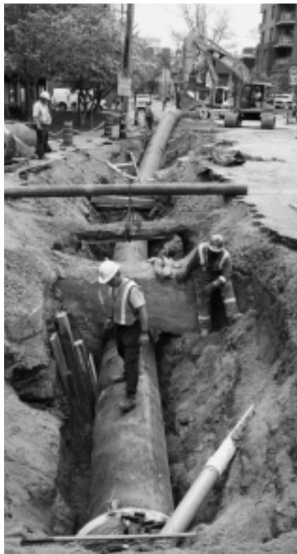
With IRC's patented non-destructive test method, municipalities can avoid the typical disruption shown here, which occurs when pipes have to be accessed for inspection.
