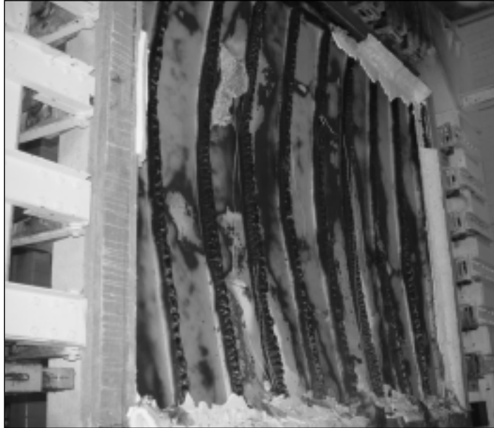
A wood-stud wall buckles during a fire test.
