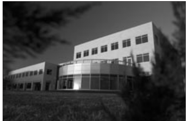
The NRC-IRC Centre for Sustainable Infrastructure Research (CSIR) is now up and running in a building adjacent to the University of Regina campus, to facilitate the free flow of staff, and ideas. Photo courtesy of Saskatchewan Research Council
