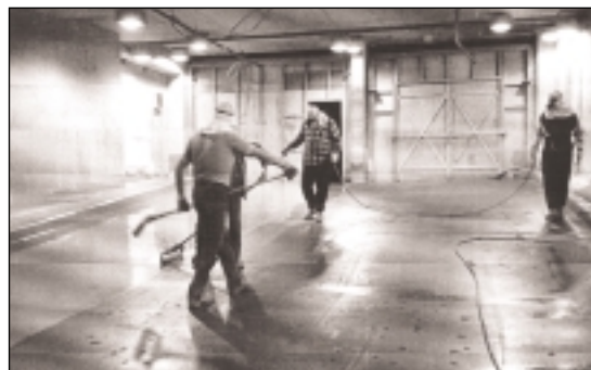
Figure 1. Application of an elastomeric waterproofing membrane system by spraying and back rolling
