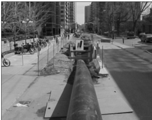
Figure 1. Watermain slipline rehabilitation, Gloucester Street, Ottawa
