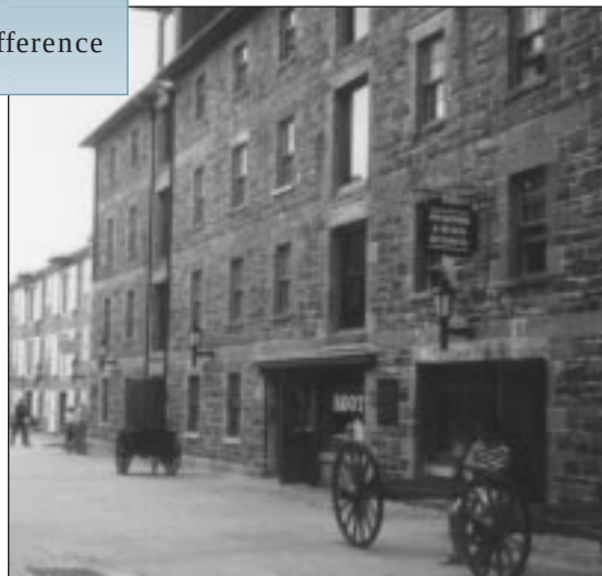
Figure 1. Massive masonry construction
