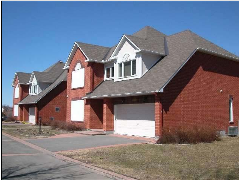
Figure III-3.1 : CCHT Twin-House Facility - with 2 south windows shaded to reduce passive solar gains.
