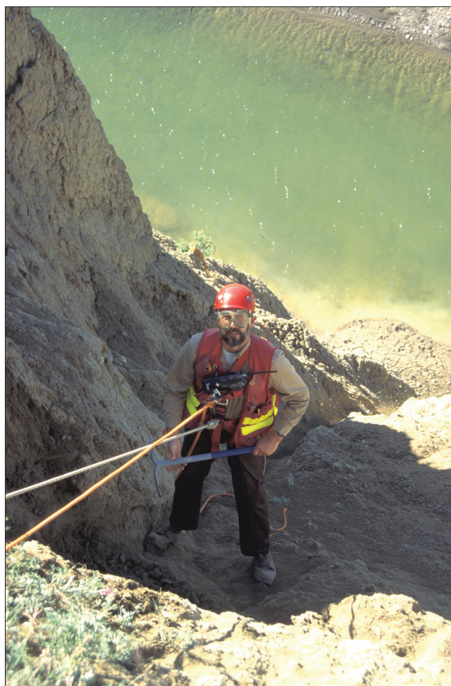
Figure 8. Two-rope system used for investigation of near vertical cliff-bank sections. Upper rope at chest is a rappel rope under the control of investigator. The lower rope is a belay rope under the control of a belayer located at the cliff top. Each rope is fixed to a separate anchor system. A two-way radio (antenna at shoulder) allows communication with belayer who takes notes and raises and lowers samples. GSC 2003-295
