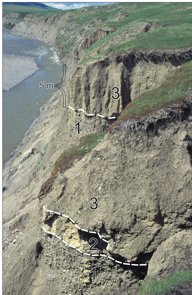
Figure 12. Succession of bouldery cobble gravel (unit 1) overlain by glaciolacustrine sediments (unit 2) and montane till (unit 3) above Oldman River (base of section O11). Unit 2 has been intensely sheared by the passage of ice that deposited unit 3. GSC 2003-299
