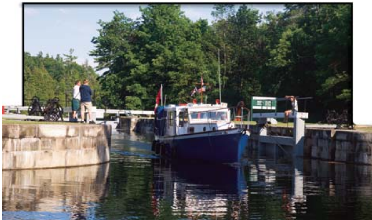
Davis Lockstation, Rideau Canal National Historic Site of Canada (ON), © Parks Canada, PHOTO: A. Guindon
