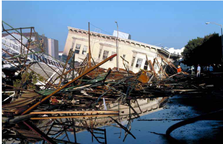
Figure 2.4.3.1-1 Examples, From Recent California Earthquakes, of How Earthquakes Can Seriously Damage Residential Property and Transport Infrastructure. [Source: United States Geological Survey]
