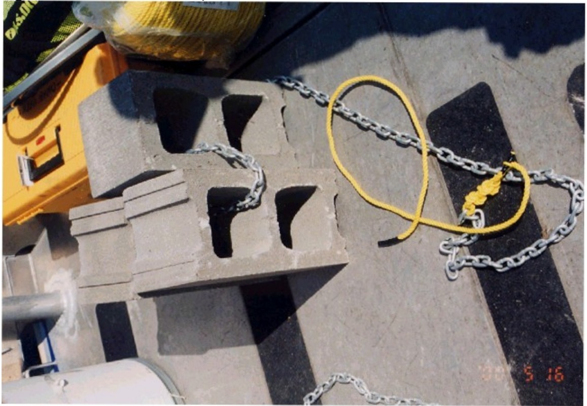
Figure 7. Concrete block set up
