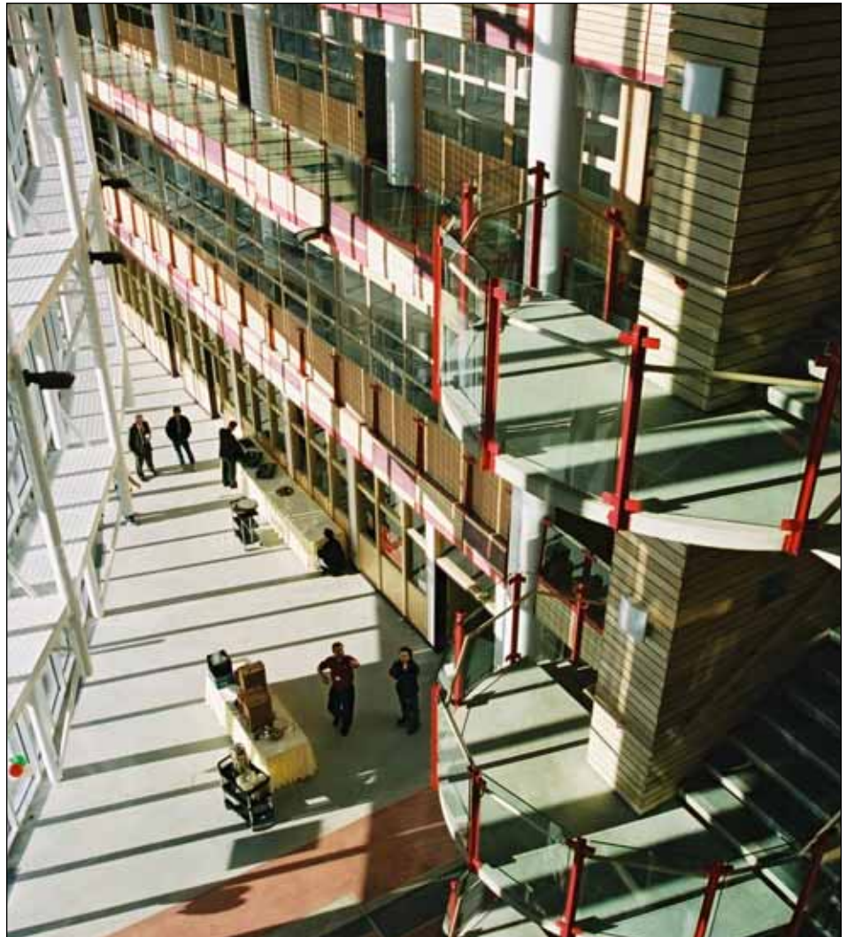
The main foyer of The Greenstone Building in Yellowknife gets natural light from the curtain wall of windows. The exterior curtain wall is equipped with solar panels.
