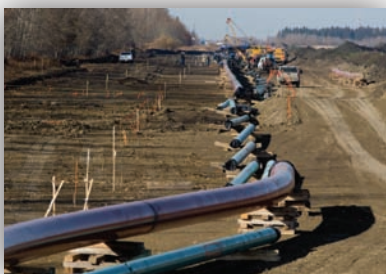
Waupisoo pipeline construction in October 2007
