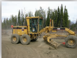
Grader on road maintenance project for Husky Energy
