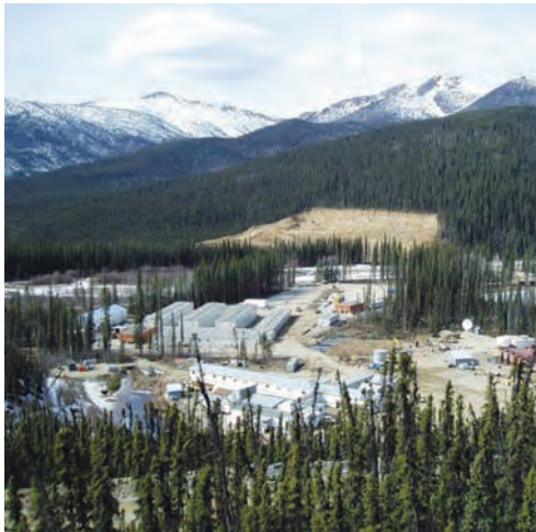
A typical ESS Support Systems remote location facility
