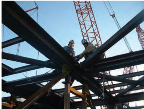
Steel erectors at work
