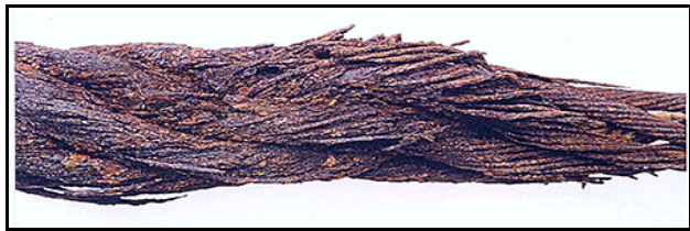
Photo 4. Port lashing cable
