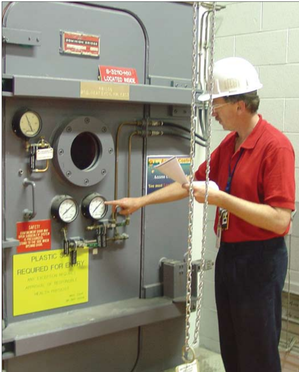
CHECKING THE CONFINEMENT DOOR TO ENSURE THE SEALS ARE INFLATED AND WITHOUT LEAKS.
