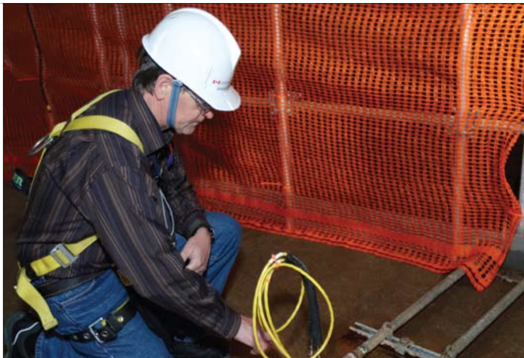
INSPECTOR CHECKING THE STATE OF COMPONENTS INSIDE THE VACUUM BUILDING.
