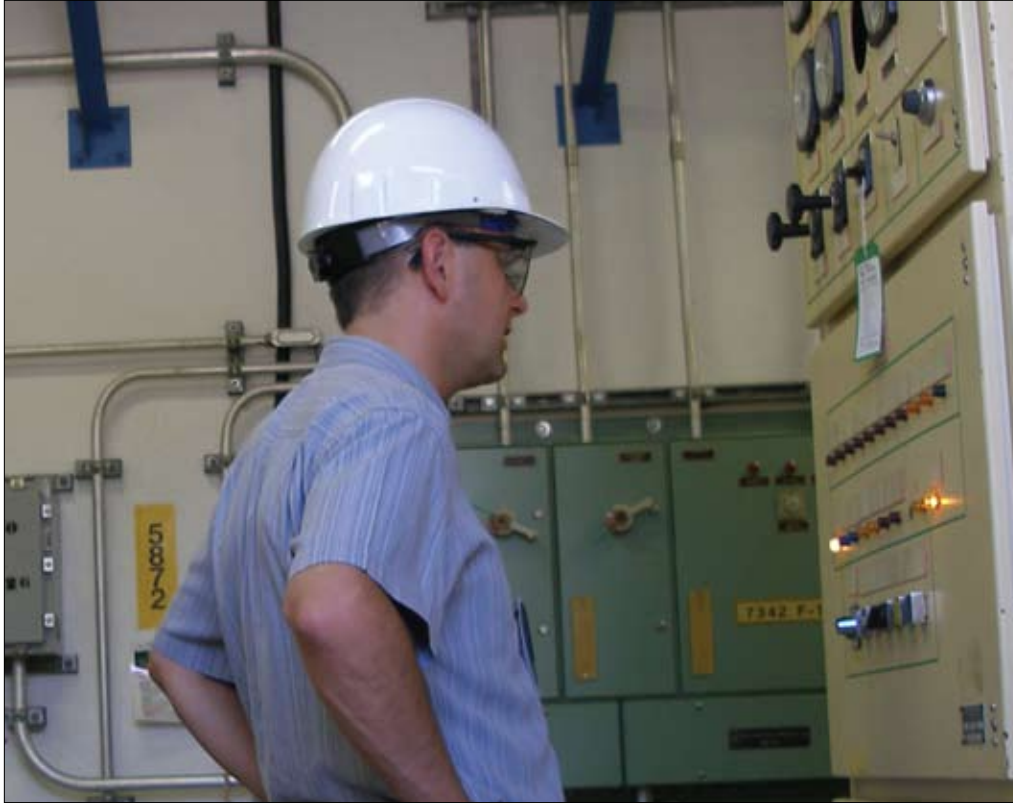
INSPECTING PANELS TO VERIFY SAFETY IMPORTANT COMPONENTS ARE READING CORRECTLY.
