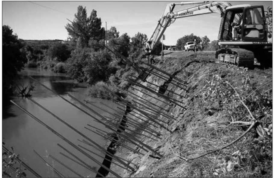
Nail shooting work in progress
