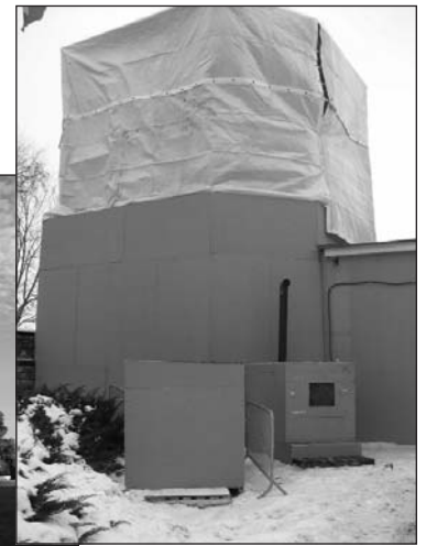
Flag pole structure on the Vaux wall of Parliament Hill (left); the same structure with heating enclosure in place following the application of fresh mortar (right).
