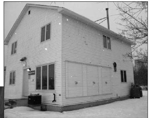
The Ventilation and Walls Research House with three identical side-by-side wall specimens
