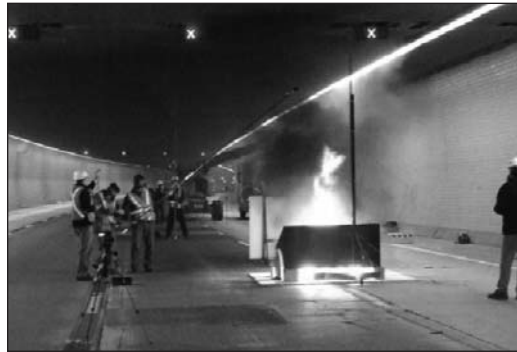
Fire detection experiments being conducted in the Carré-Viger Tunnel in Montréal.
