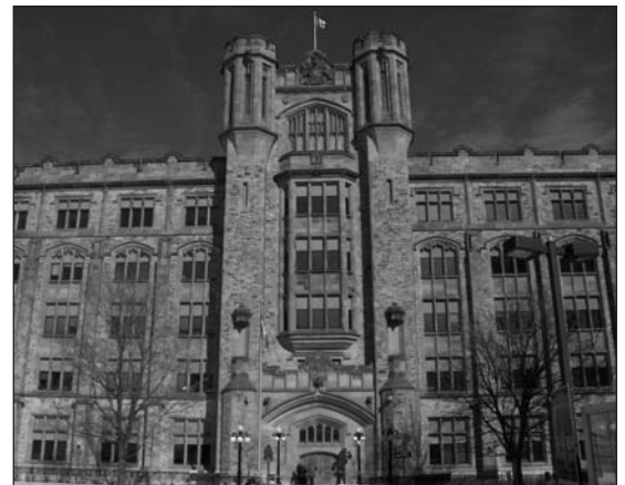
Figure 1. The Connaught Building in Ottawa, built in 1913-14, is clad with Nepean and Wallace sandstone, with granite at grade.
