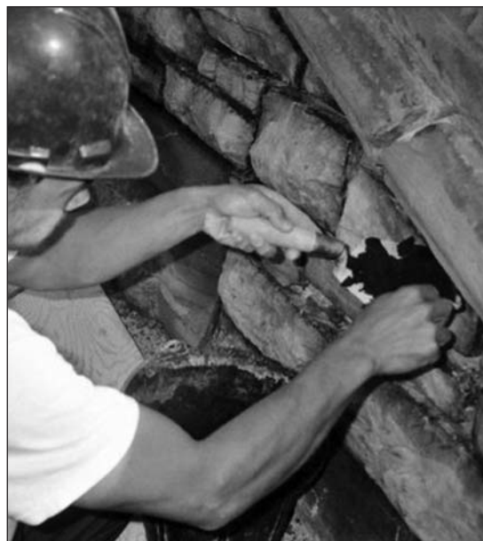
Figure 1. Repointing is the process of removing the outer (deteriorated) layer of mortar and replacing it with new mortar.
