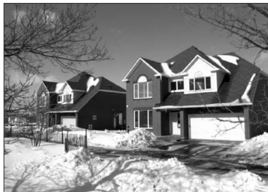
Figure 2. The Canadian Centre for Housing Technology is operated as a partnership between NRC, Canada Mortgage and Housing Corporation, and Natural Resources Canada.
