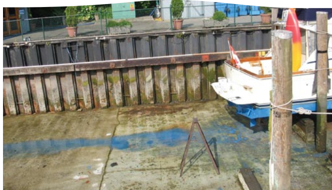
Example of a boat being powerwashed on a tidal grid facility that has a collection system for anti-fouling paint waste
