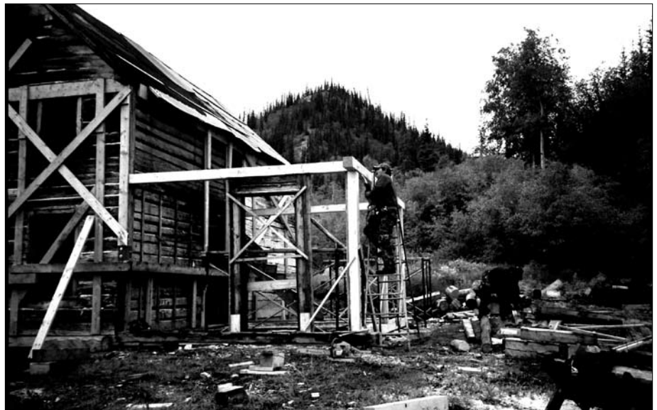
Crew working to restore Cadzow House kitchen.
