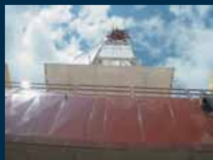
Drilling rig on Stoney Nation lands, Alberta.
