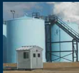
Oil tanks at O'Chiese First Nation, Alberta.
