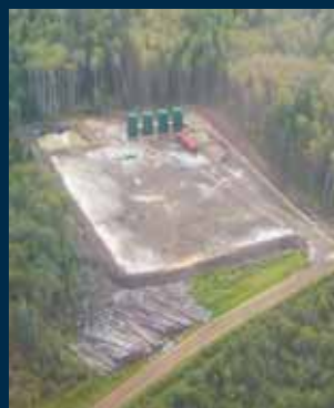
Construction of surface site on Bigstone Cree Nation lands, Alberta.
