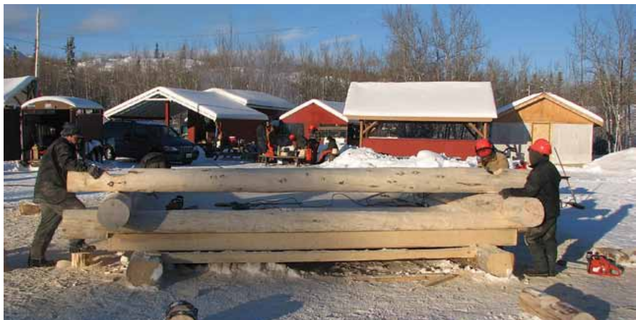
Scribing is the process of marking a log to fit the log below it. Students shown here are learning the skill as part of the 2008-2009 Log Building Training Program hosted by the Ta'an Kwäch'än Council and the First Nation of Na-Cho Nyäk Dun. For more information contact the Training Policy Committee at 867-668-7812.
