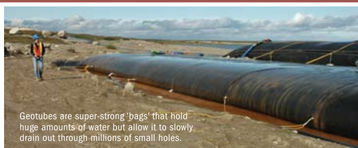
The water inside the bag gets forced through the holes by its own pressure and the contaminants stay inside.
