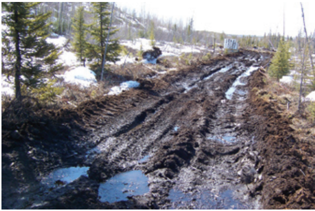
FIGURE 9. Proper scheduling of road construction will avoid rutting and erosion.
