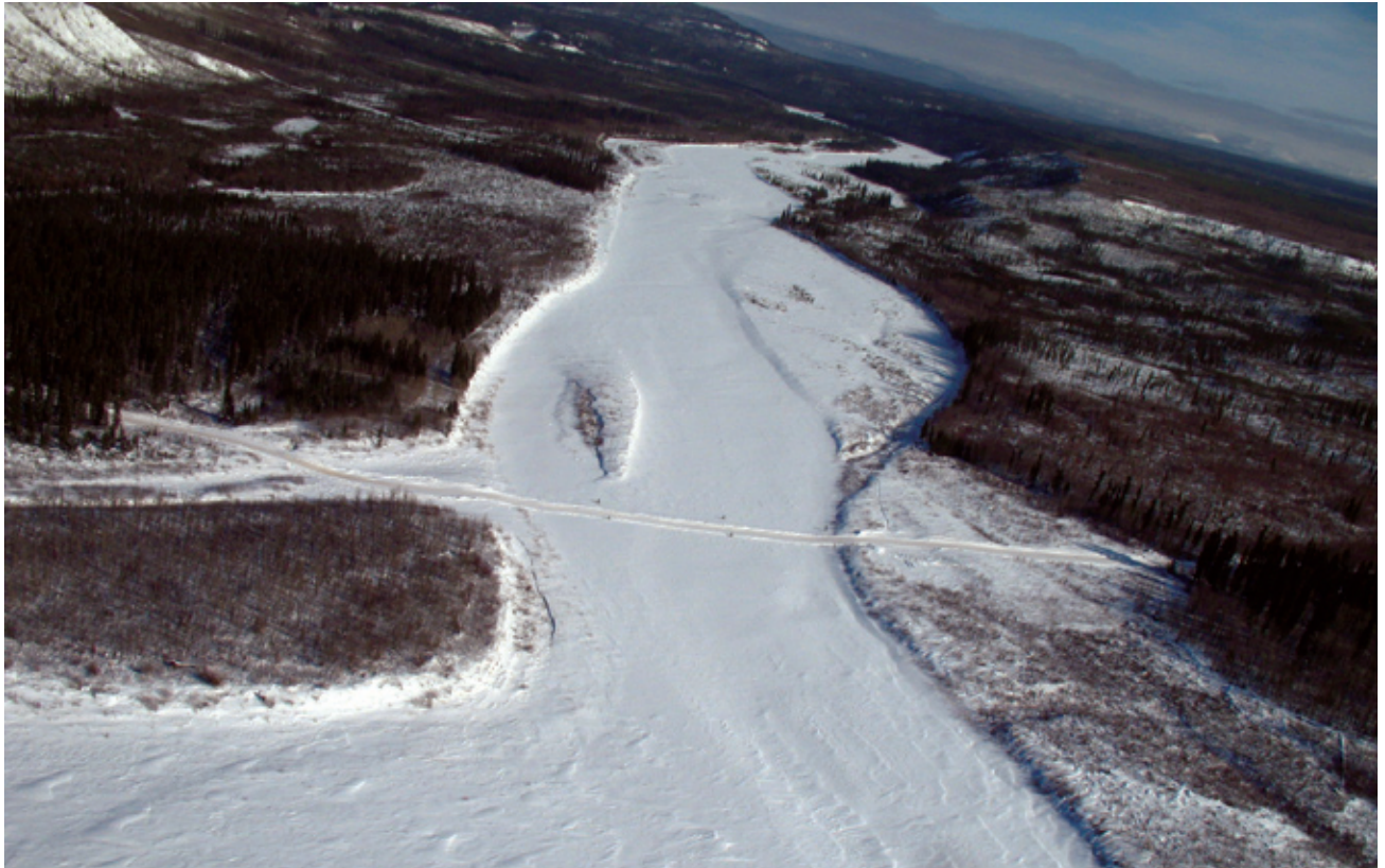
FIGURE 35. An ice bridge built over a large stream channel.
