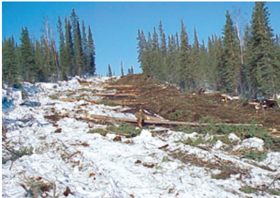
FIGURE 14. Brush can be used as a sediment trap on steep slopes.
