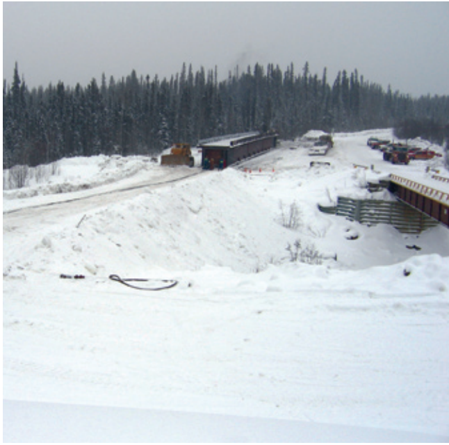
FIGURE 33. A well-constructed snow fill located adjacent to a new bridge.
