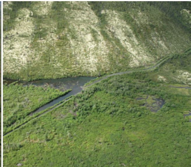
FIGURE 3. Field investigations should be conducted in both the summer and the winter to ensure that the road is built with consideration for the full range of climatic and hydrological conditions.
