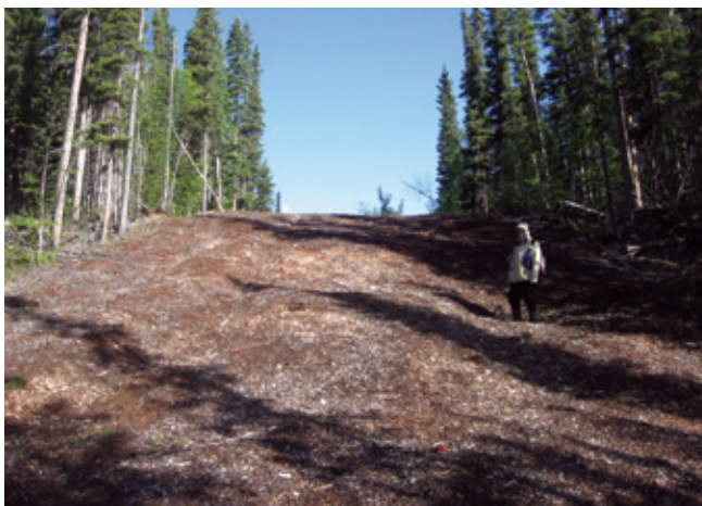
FIGURE 40. Differential settlement can occur in ice-rich permafrost terrain.
