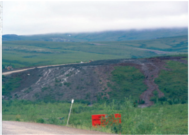
FIGURE 39. Regular monitoring will identify areas where drainage controls are inadequate and need to be redesigned.
