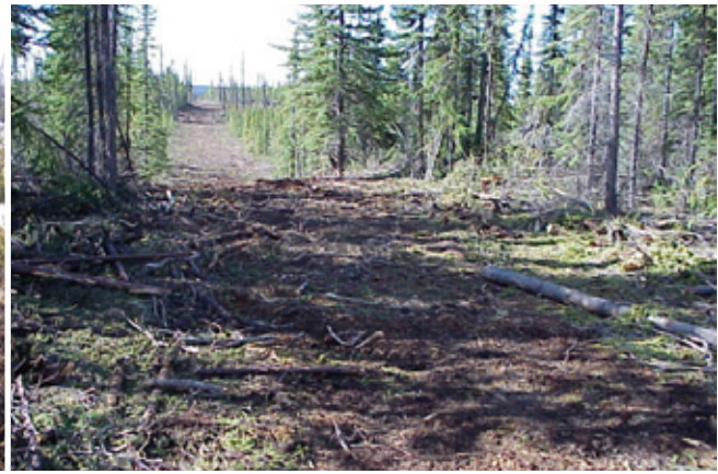
FIGURE 10. Clear only the minimum width necessary for road use.
