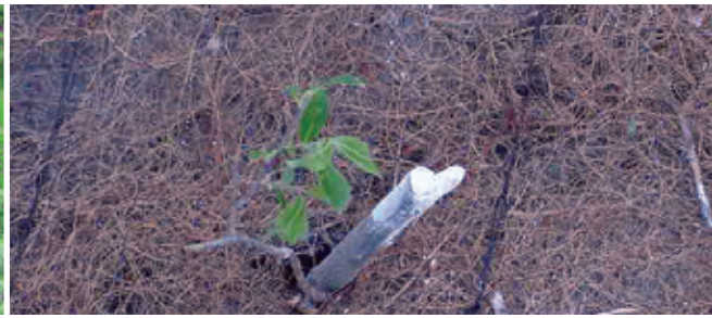
FIGURE 45. Erosion control can include the use of mats and planting willow cuttings.
