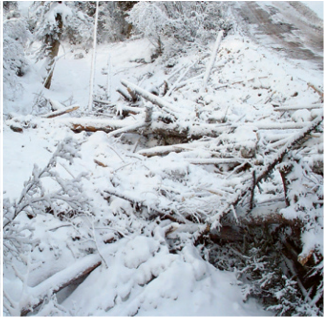
FIGURE 34. A poorly constructed snow fill consisting of mixed brush and snow.
