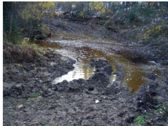
FIGURE 24. Fording of this stream has resulted in rutting, sedimentation and erosion of the channel banks.
