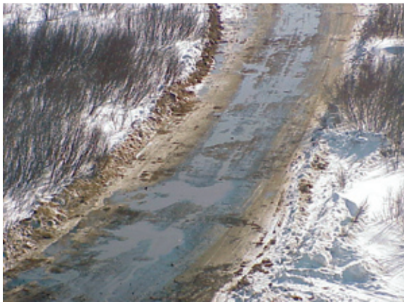
FIGURE 31. (Top) Winter roads are not ready for use by heavy wheeled vehicles until there is at least 10 cm of packed snow. Visible grass on this road indicates that there is less than 10 cm of snow.
