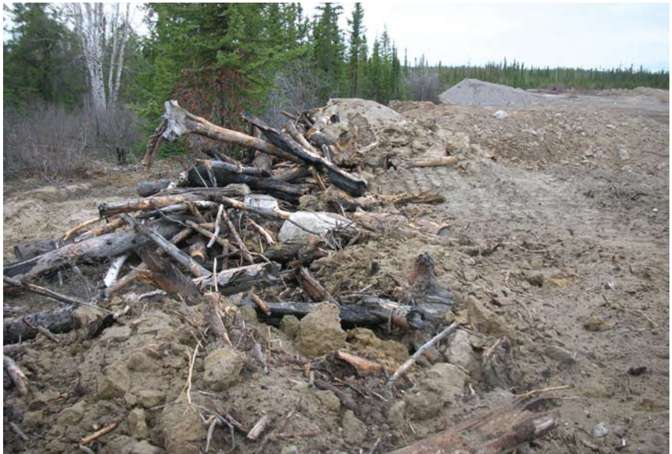
FIGURE 20. Overburden and woody debris should not be mixed, and piles should be at least 5 m from standing timber.
