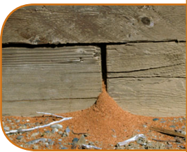
Sawdust shavings ejected from a carpenter ant nest Photo: Edward H. Holsten, USDA Forest Service, Bugwood.org
