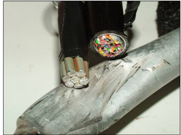
Photo 2. Cable markings on crankcase vent tube
