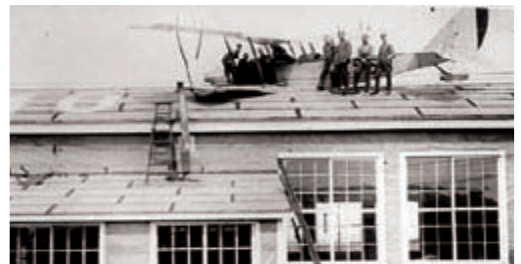
Damaged Curtiss JN-4A(CAN) aircraft C568 of the Royal Air Force on the roof of a hangar. Library and Archives Canada / PA-102835
