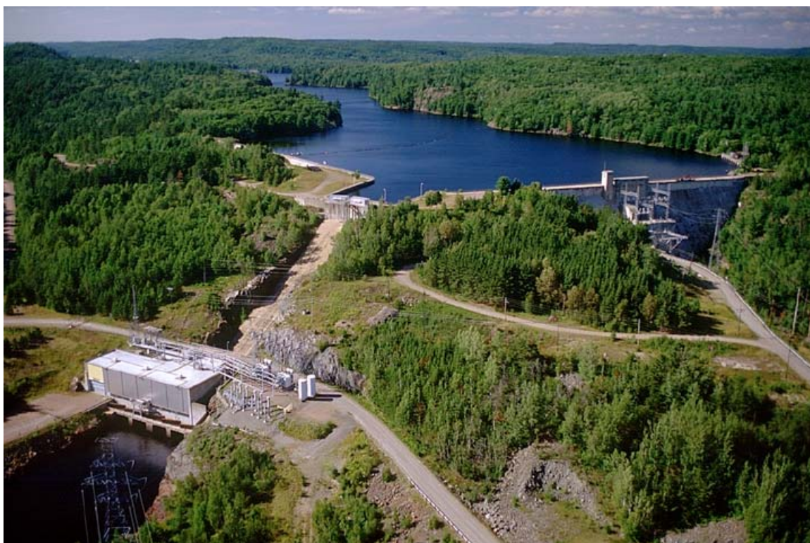
Wells Generating Station on the Mississagi River at Wharncliffe, Ontario. Photo Courtesy of Brascan Power Corporation.
