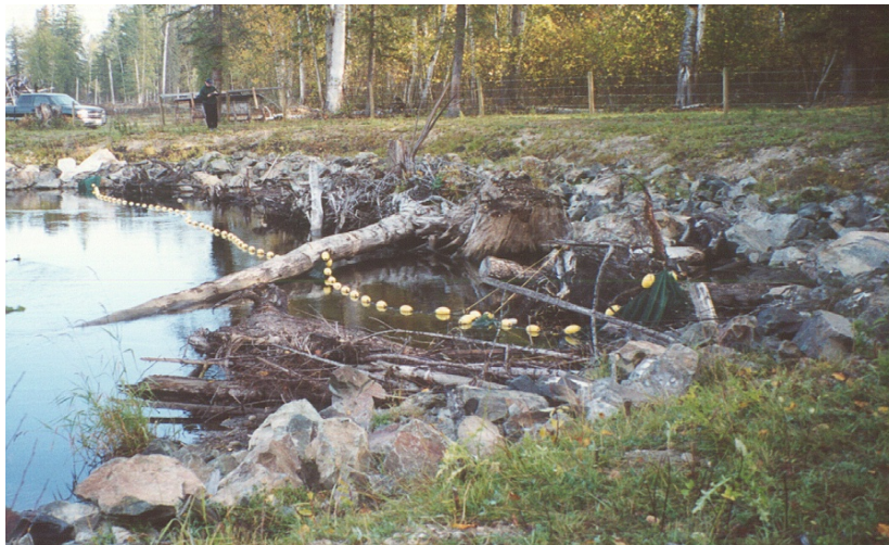
Figure 18: Good habitat value provided by rip-rap and large woody debris on Mann Creek.
