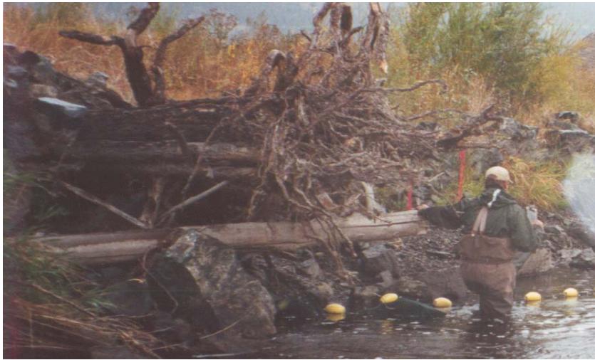
Figure 19: Elevated rootwad placement provided limited fish habitat value.
