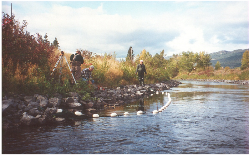
Figure 17: Typical rip-rap bank protection on the lower Nicola River.
