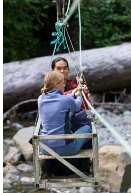
Cable car, Cullite Creek on the West Coast Trail. Parks Canada/J. McCulloch
