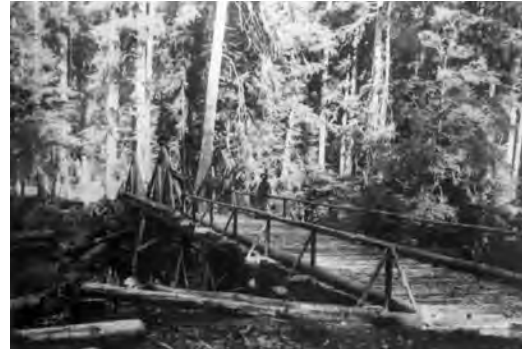
Trestle near Pachina Point, West Coast Lifesaving Trail. Dept. of Transport Marine Division Collection, Victoria
